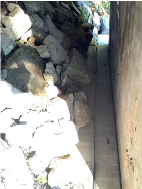
Left Bank Abutment when facing downstream
