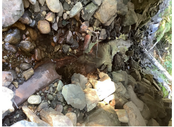
Old boiler culvert left in place
