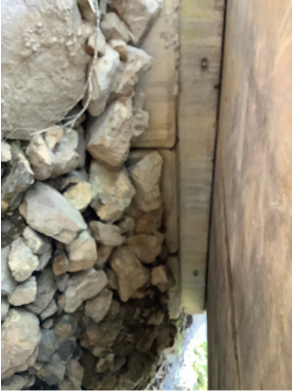
Right Bank Abutment when facing downstream
